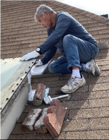
Willie Lew repairing skylight
