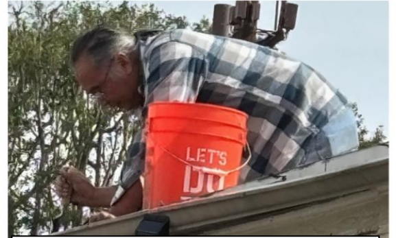
Gordon Hom cleaning gutter at CHSSC
